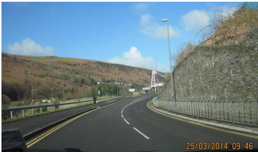
Figure F4: Northbound view in the southern section of the link
